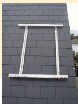
Figure 13 – Installed Roof Bracket
